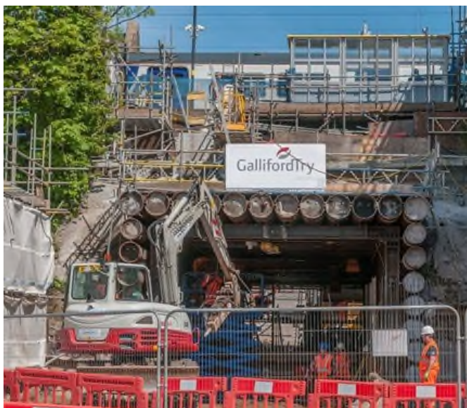
Construction-stage reference photograph from the original project archive. Galliford Try site shown.
