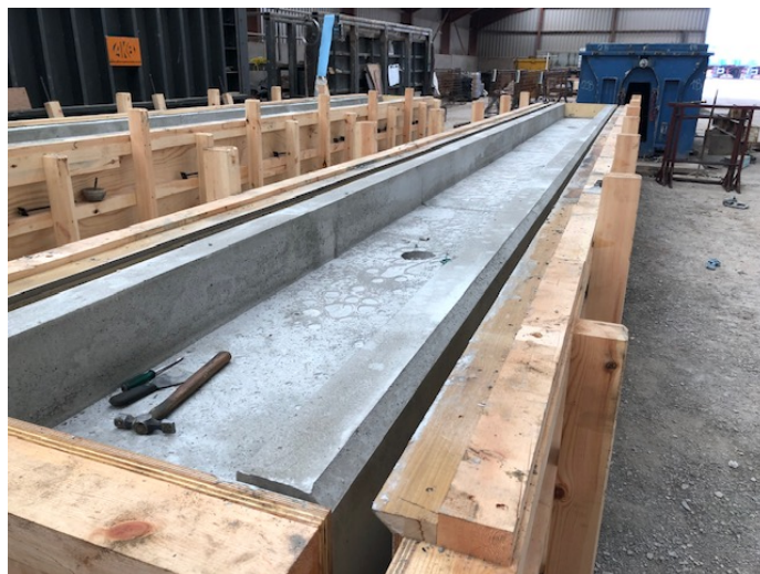
Precast capping beam during manufacture. Bespoke units were developed to suit the surveyed wall alignment.
